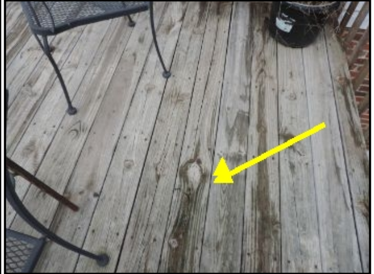
Grounds Patio and Porch Condition
