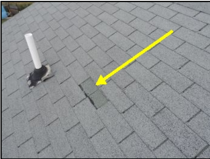
Roof Roof Condition
