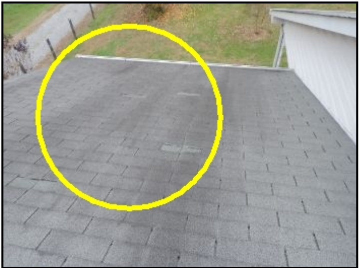
Roof Roof Condition
