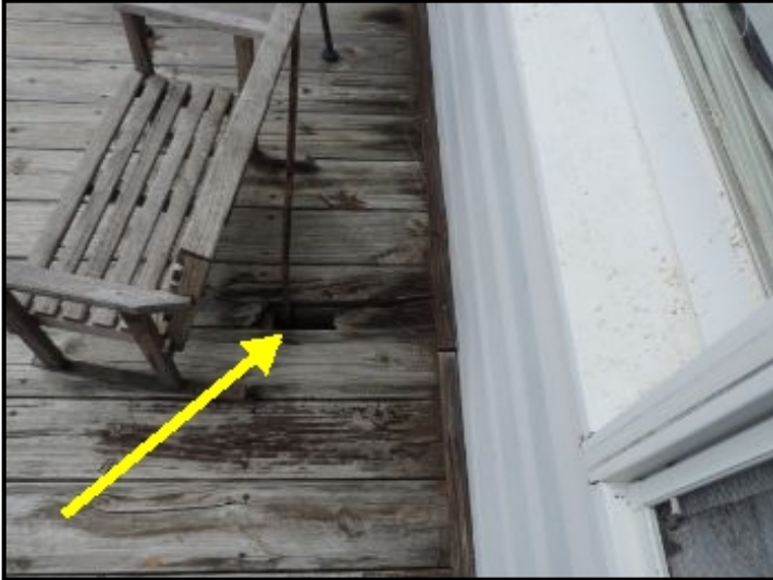
Grounds Patio and Porch Condition
