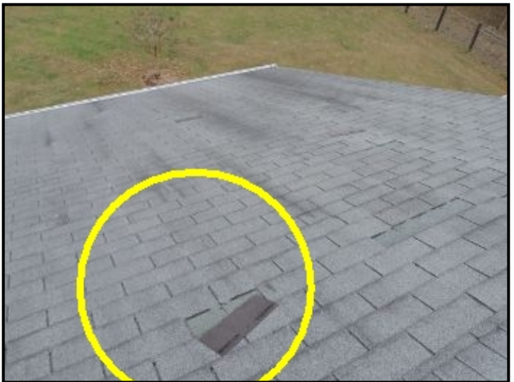
Roof Roof Condition
